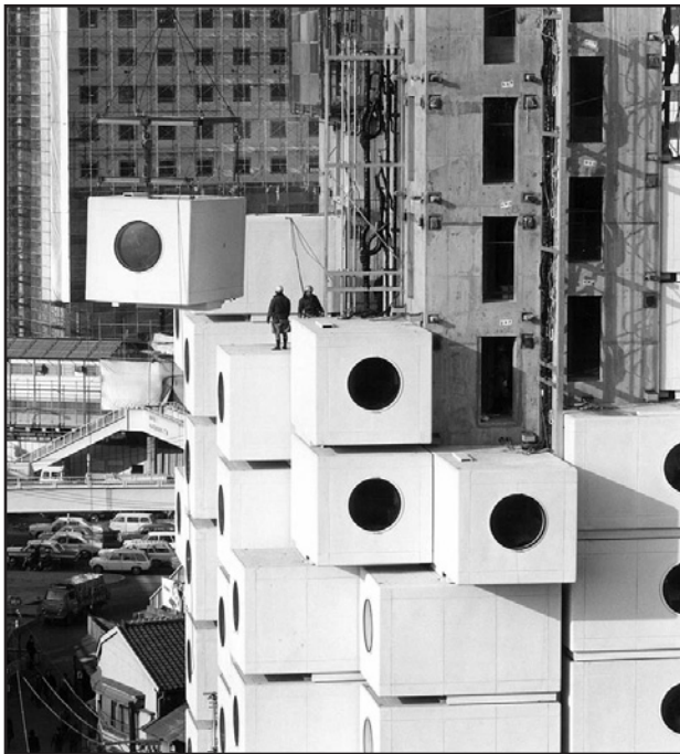
Fig. 6 Construction of Nakagin Capsule Tower
