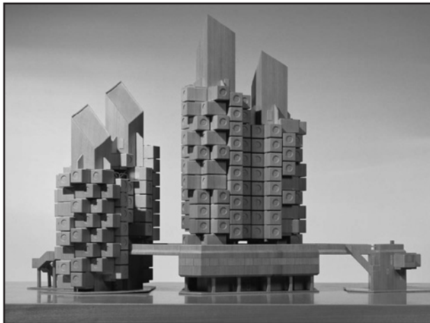
Fig. 4 Model of Nakagin Building indicating possibility of expansion
